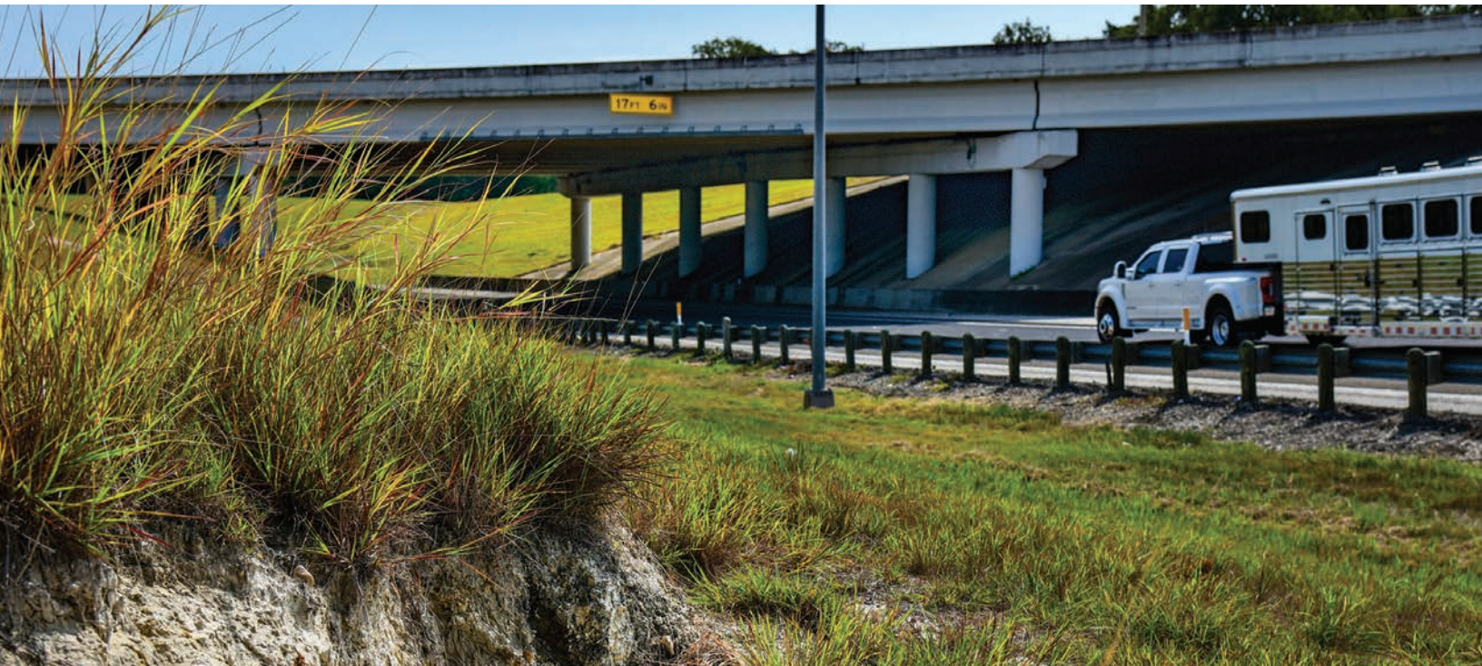
TTI researchers evaluated methods for protecting the area near a roadway, shown here, from uncontrolled erosion.
